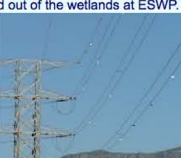
Powerlines over the retention dam at Edith Stephens Wetland Park (ESWP) cause the death of birds that collide with them.
