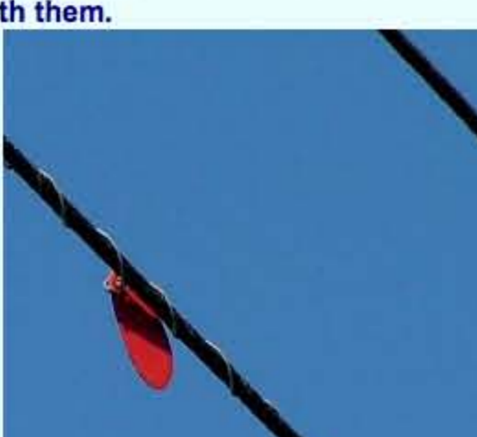
'Bird flappers' have been attached to the cables to make them more visible to the birds.
